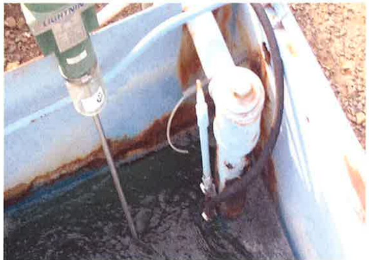
Photo 6 – Existing Return Activated Sludge Piping System
